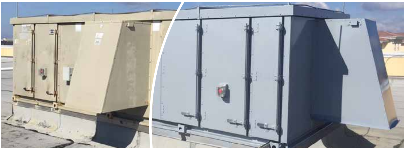
AHU Roof Top Unit After HVAC New Life
